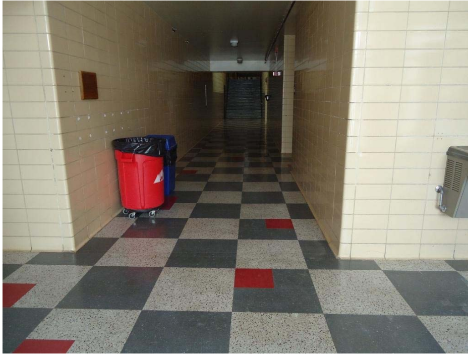
Photo 3 – View of Flooring in Main Hallway. Floor Tile – ND, Mastic 4% Chrysotile.
