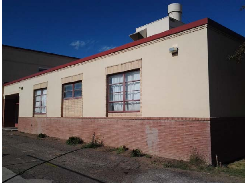
Photo 5 – View of Exterior Windows to be removed during Phase I.
